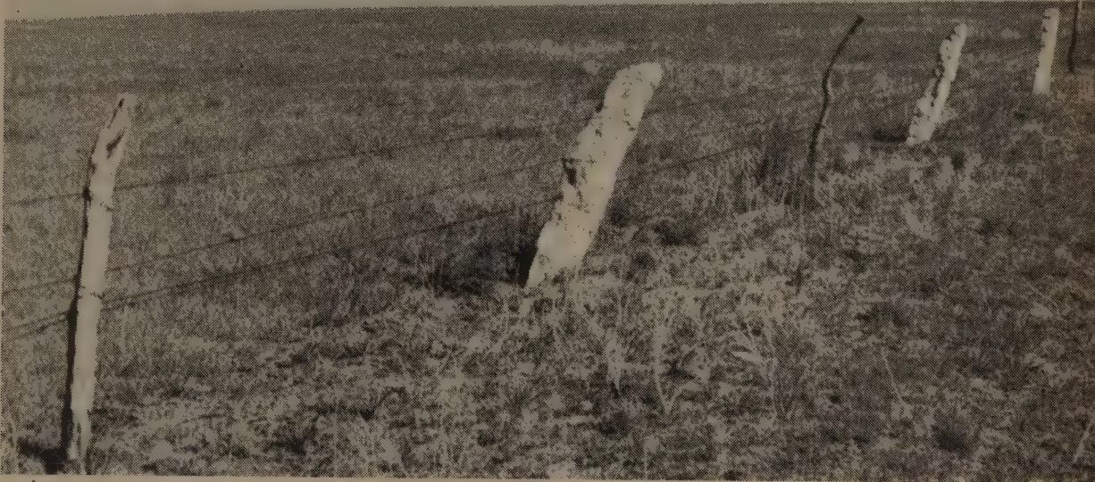
Barbed wire made possible the settlement of the Great Plains and, in this treeless land, limestone fence posts made possible barbed wire.
